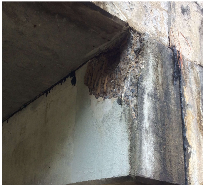
PHOTO 4 Description Cap - Bent 37 right: Spalling
