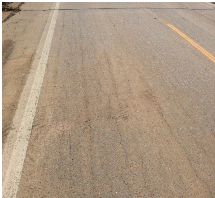
PHOTO 1 Description Span 16 large unsealed longitudinal crack.
