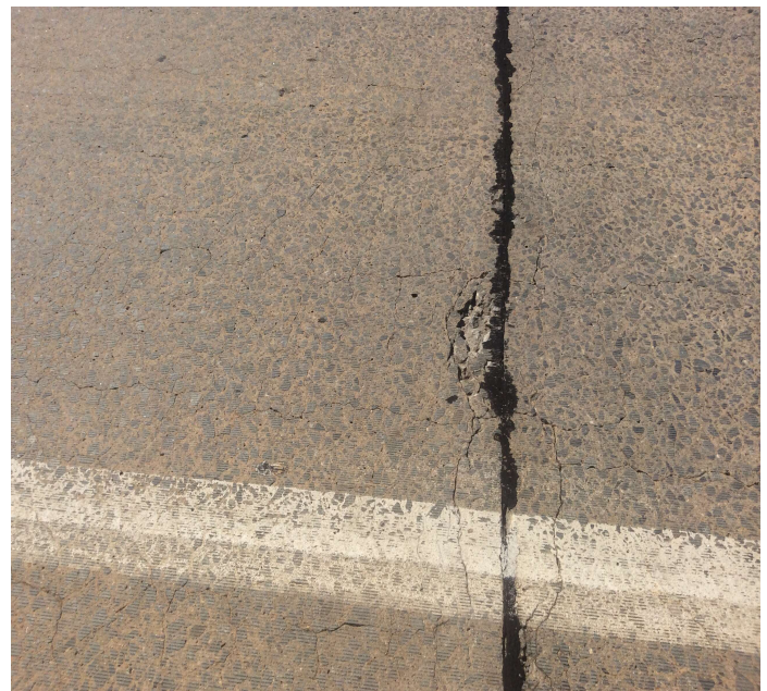
PHOTO 2 Description Span 29 at bent 29 left lane small spall forming at joint.
