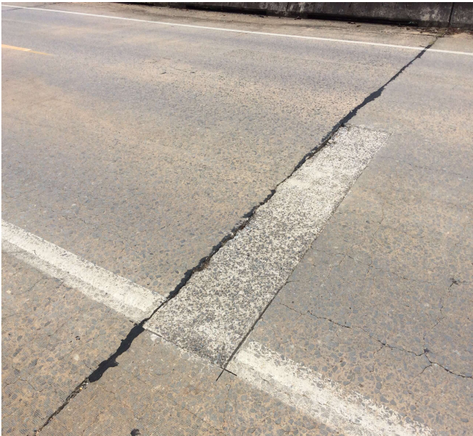
PHOTO 4 Description Deck - Bent 25 left: Patch deterioration
