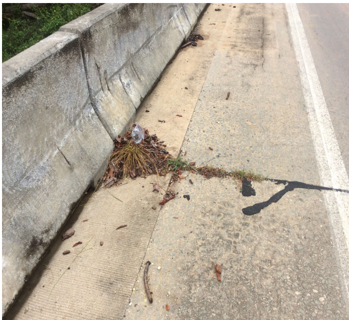
PHOTO 3 Description Gutterline/joint - Bent 16 left: Vegetation/debris build-up
