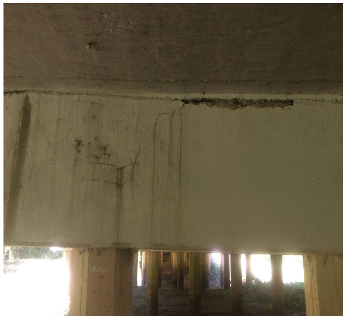
PHOTO 1 Description Bent 6 ahead cap over pile 5 cracked and Delams.
