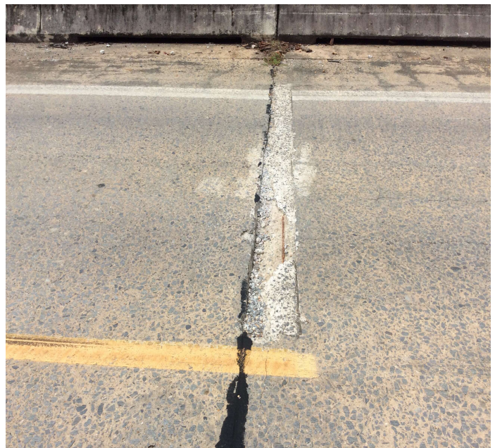
PHOTO 2 Description Deck - Bent 21 right: Patch deterioration
