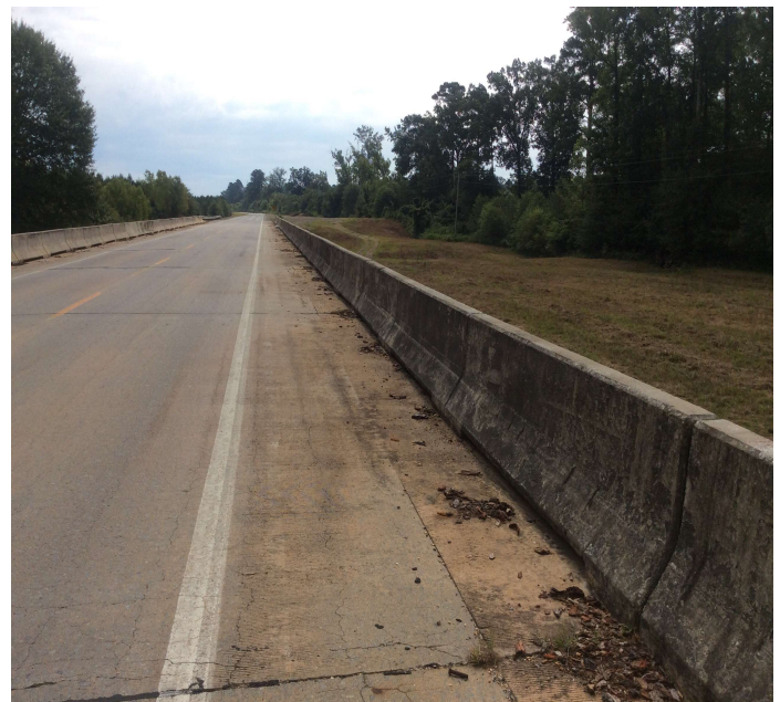
PHOTO 2 Description Gutterline - Spans 28-38 right: Minor debris build-up
