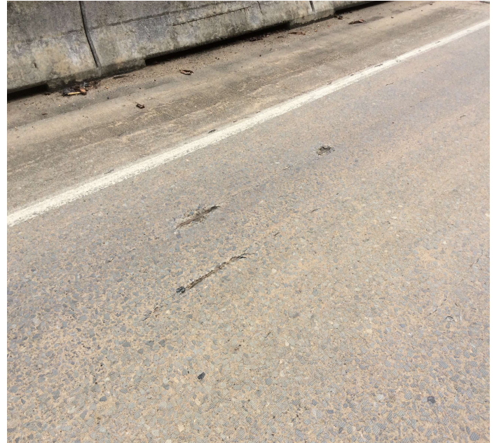
PHOTO 5 Description Deck - Span 12 left: Rebar exposed
