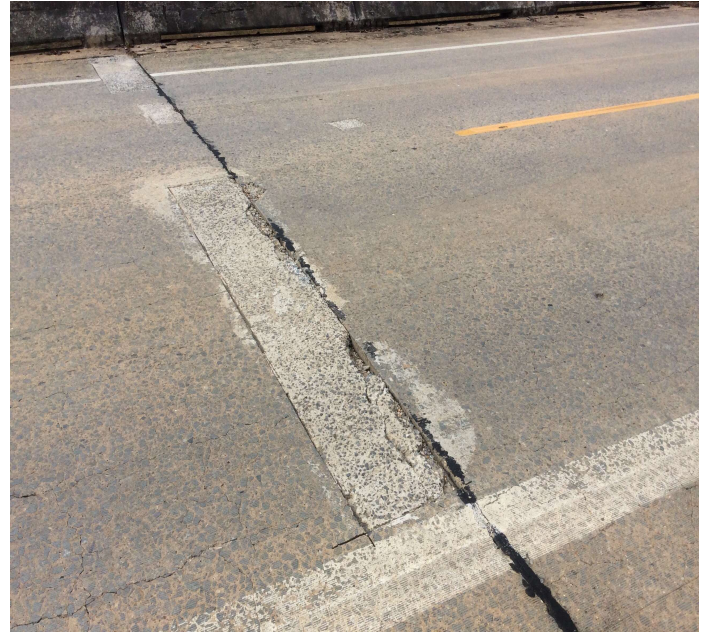
PHOTO 5 Description Deck - Bent 35 left: Patch deterioration
