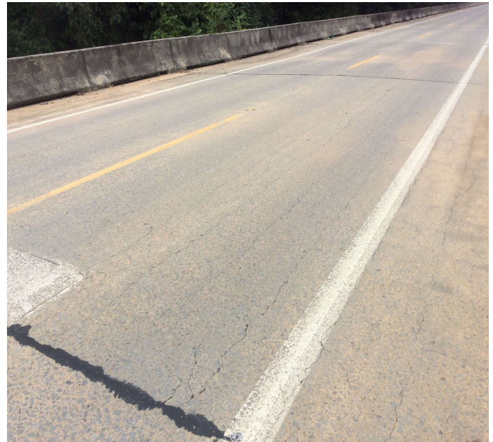
PHOTO 6 Description Deck - Span 26 left: Cracking
