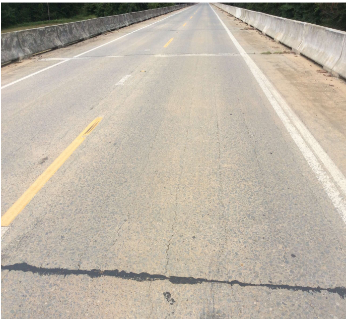
PHOTO 8 Description Deck - Span 35 left: Cracking
