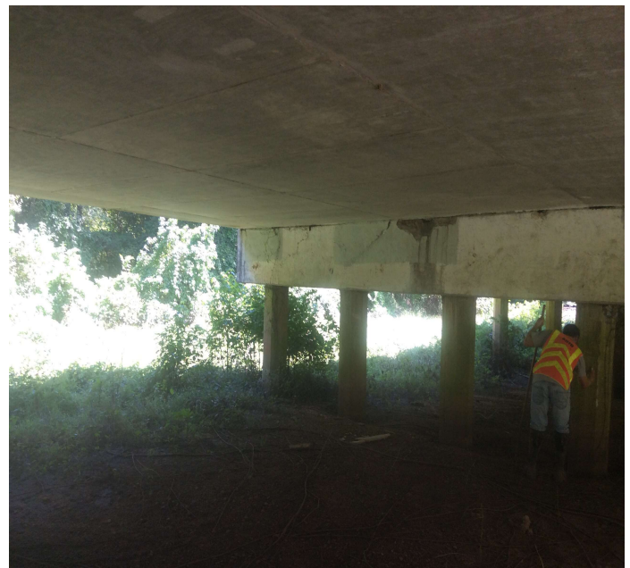
PHOTO 2 Description Bent 11 cap back spalls and Delams.
