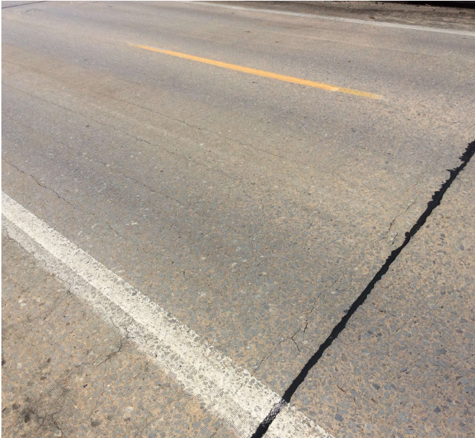
PHOTO 3 Description Deck - Span 22 left @ Bent 22: Cracking
