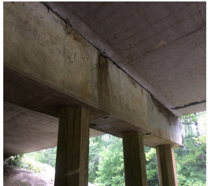
PHOTO 6 Description Cap - Bent 2 left ahead: Rebar exposed
