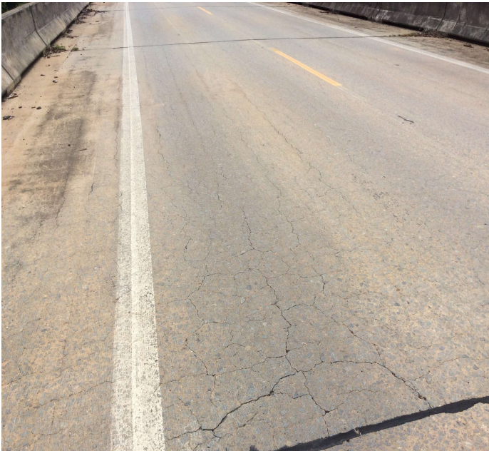
PHOTO 4 Description Deck - Span 16: Cracking
