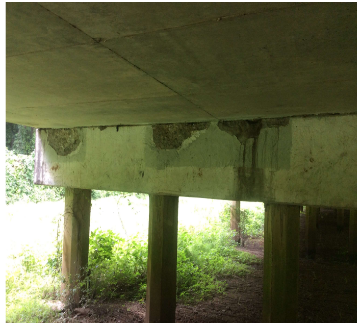
PHOTO 5 Description Cap - Bent 11 left back: Spalling
