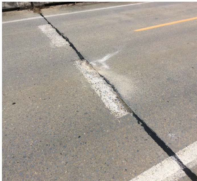
PHOTO 1 Description Deck - Bent 7: Patch deterioration
