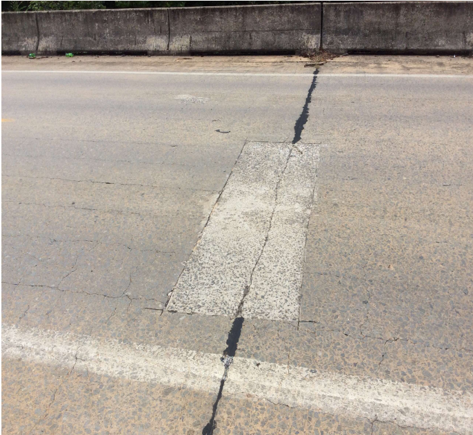
PHOTO 3 Description Deck - Bent 24 left: Patch deterioration
