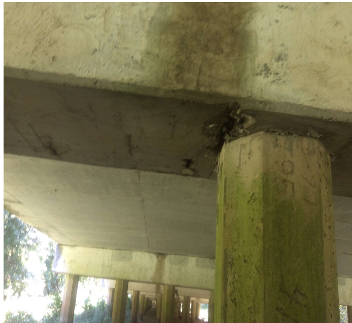
PHOTO 3 Description Bent 13 bottom of cap at pile 3 spalls with exposed rebar.
