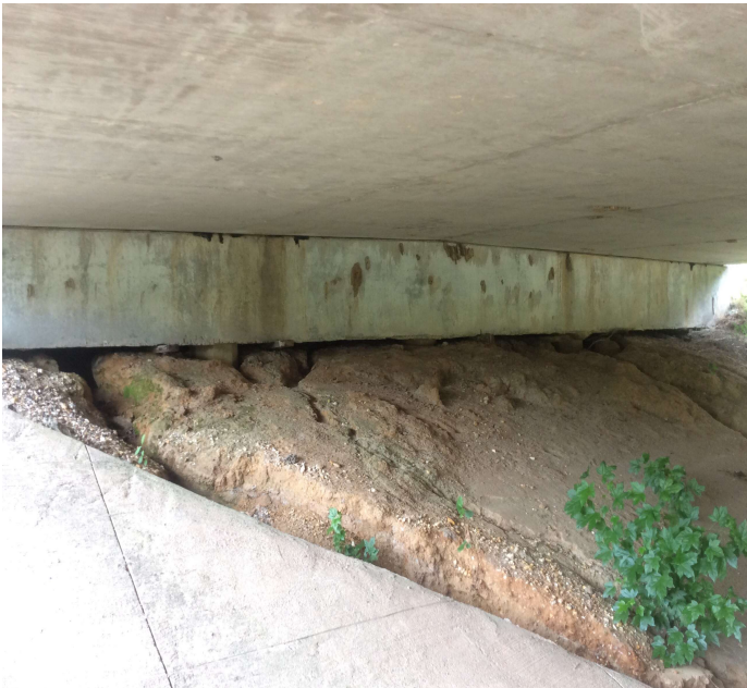
PHOTO 1 Description Endslope - Bent 38: Erosion
