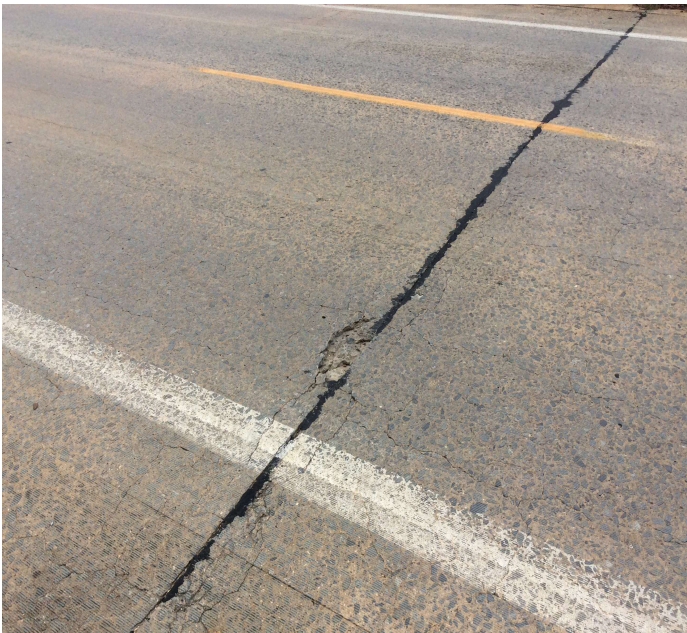
PHOTO 7 Description Deck - Span 29 left @ Bent 29: Spalling
