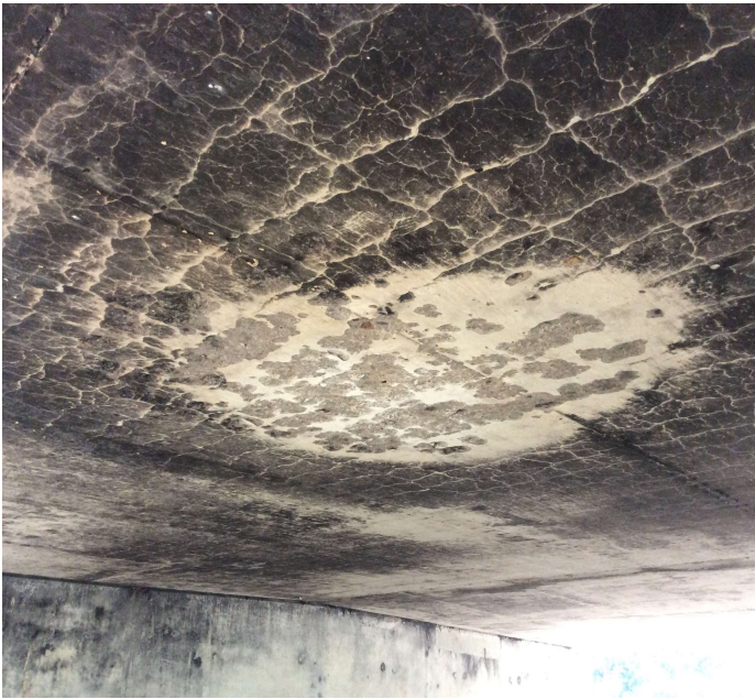
PHOTO 1 Description Soffit - Span 31 left: Fire damage
