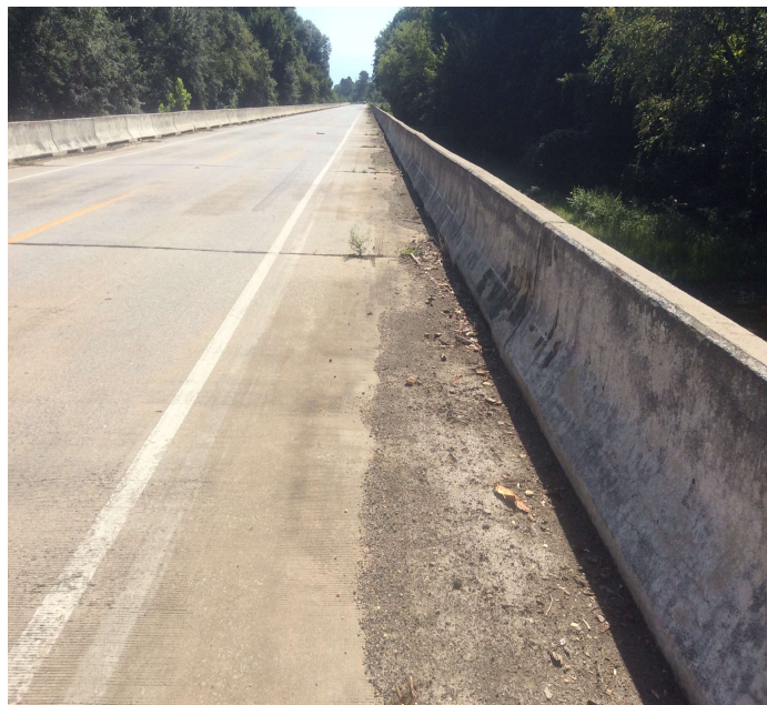
PHOTO 1 Description Right gutter line debris.
